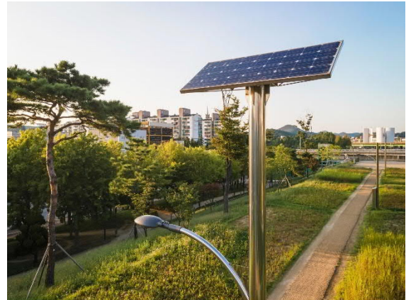
Figure 1 - Solar column lighting
