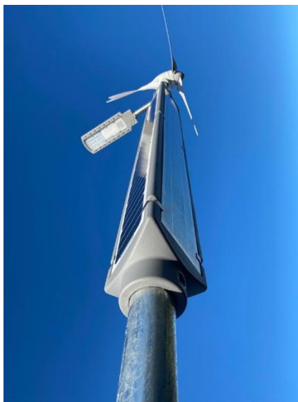
Figure 2-8 - Solar PV panel and wind turbine hybrid
